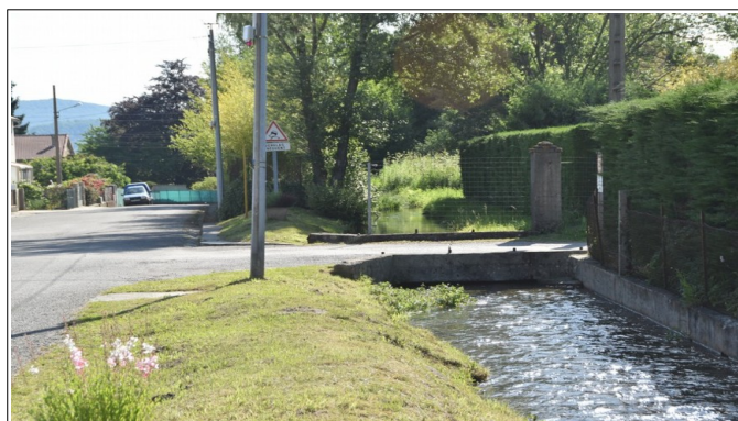
Figure 3.6: ponceau enjambant le canal.
